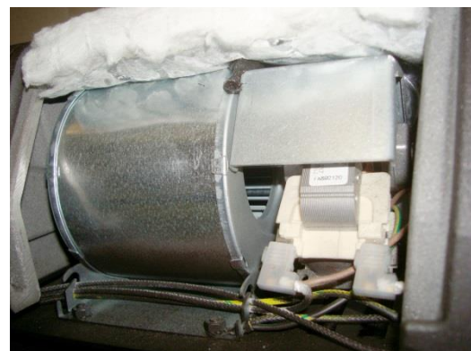
Figure No.9 - Access to fans
